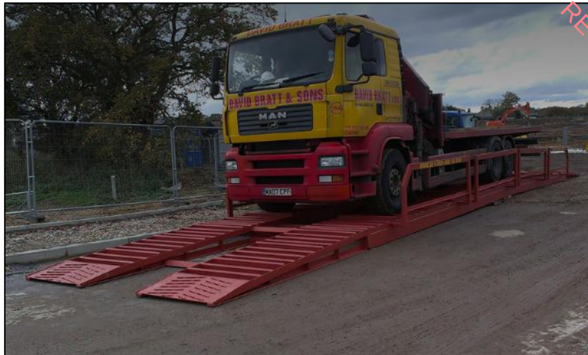
Figure 7-1 – Typical Wheel Wash
